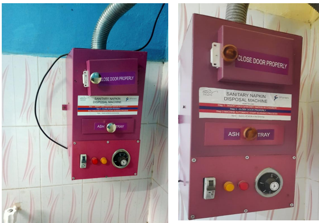
Figure 26 Sanitary pad incinerator or Sanitary napkin disposal machines located in washrooms of girls hostels and ladies toilet at college.
